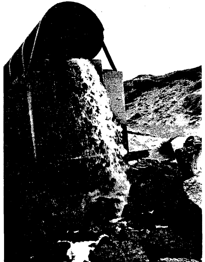
Ford Ord sewage outfall
