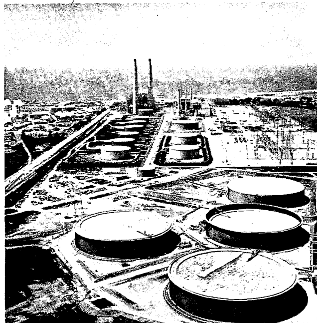
Moss Landing power plant (oil storage tanks in foreground), Monterey County
