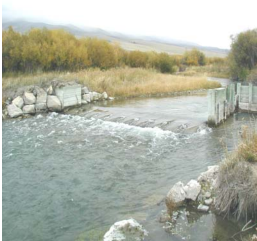
MFWP Fish Trap Facility on Red Rock River
