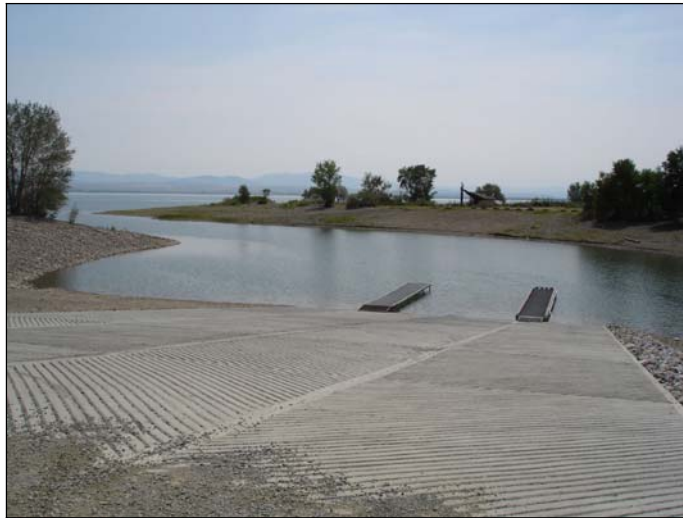
Figure 20. Silos Boat Launch Ramp
