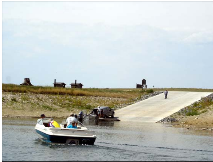
Figure 19. Goose Bay Boat Launch Ramp & Toilets
