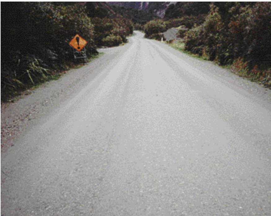
This road in New Zealand performs remarkably well because of good crown and good gravel quality in a region that receives nearly 150 inches of moisture a year! (Courtesy of Ken Skorseth, SD LTAP)
