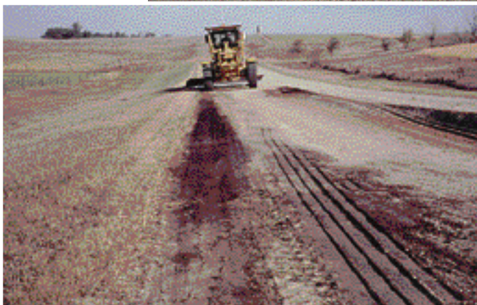
The existing secondary ditch is then cut slightly deeper and the material is placed in the roadway.
