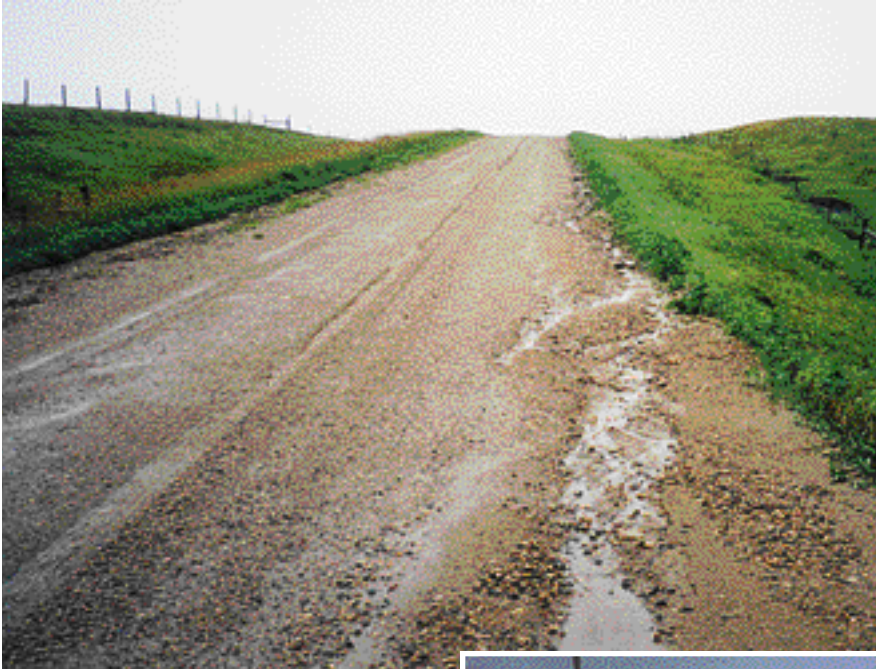
A common condition along the edge of many gravel roads: the secondary ditch.
