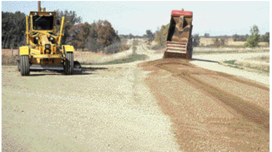
These two photos depict a the good job of spreading done by a county highway department using tandem end-dump trucks. The skill of the drivers makes this job look easy. Notice also the grader is ready to begin processing the material.
