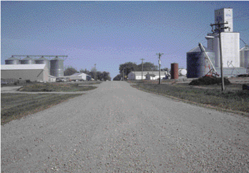
The same road as shown on the previous page approximately three months after the heavy haul was finished. The road was restored to remarkably good shape simply with the use of motor-graders doing a complete reshaping of the inslope, shoulder and surface with a small amount of surface gravel added.
