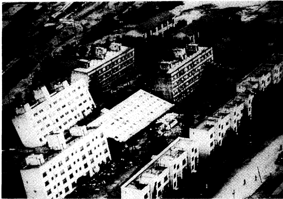
Figure 2. Tilting of buildings due to soil liquefaction during the Niigata (Japan) earthquake of 1964.
