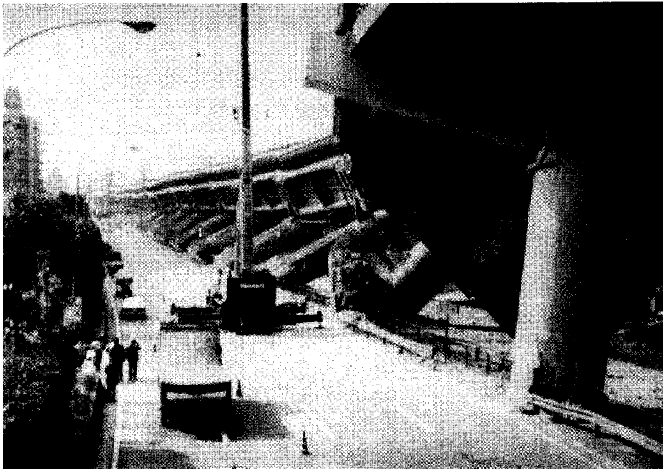
Figure 5. Collapse of Hanshin expressway during the 1995 Kobe (Hyogo-Ken Nabu, Japan) earthquake.
