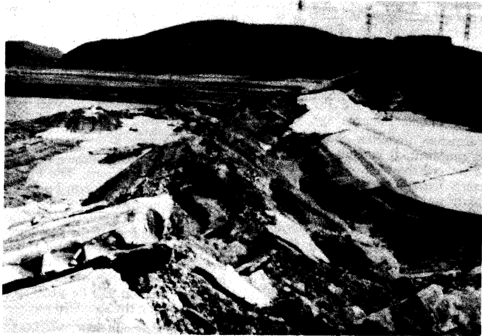
Figure 3. Slumping of the Lower San Fernando Dam in the 1971 San Fernando earthquake.
