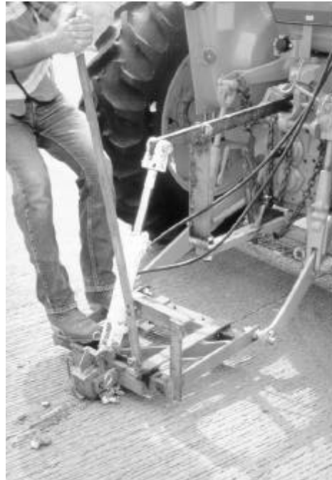
Figure 12. Joint plowing operation.
