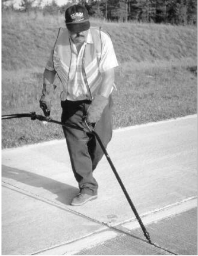
Figure 17. Hot-applied sealant installation.
