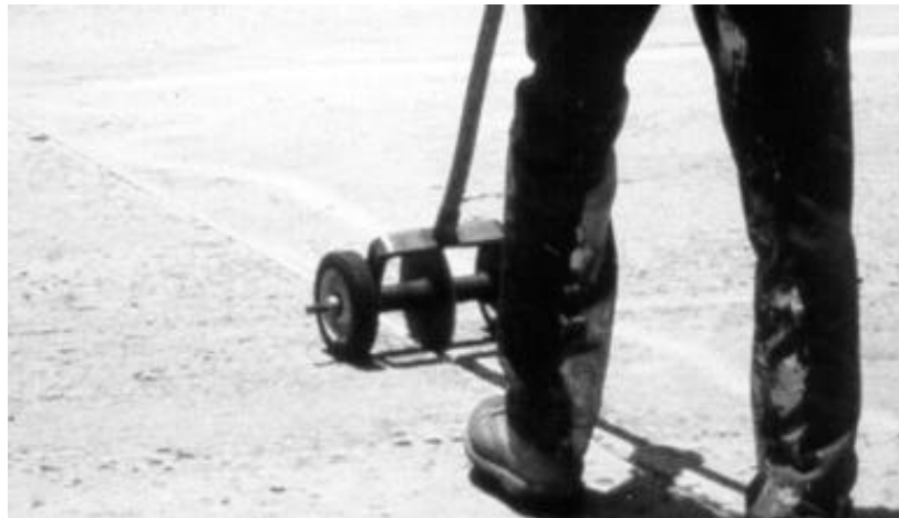
Figure 10. Hand-operated backer rod installation tool.
