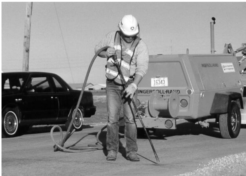
Figure 15. Airblasting operation.
