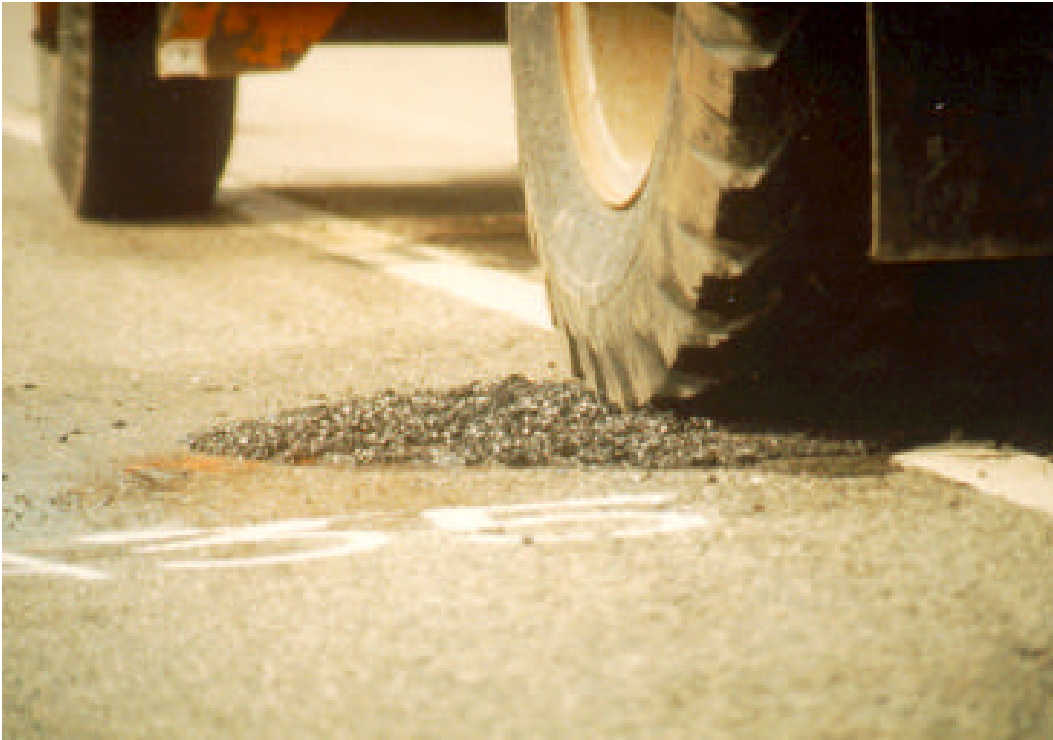
Figure 2. Throw-and-roll procedure—compaction of patch.
