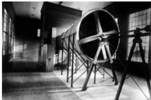
The first major U.S. wind tunnel was built at NASA’s Langley Research Center; Hampton, Virginia in 1920.
