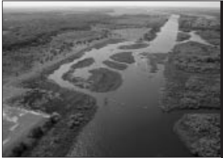
Kissimmee River canal and test fill
