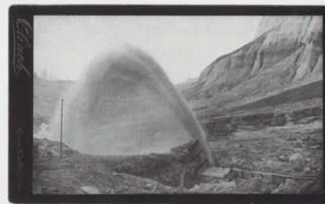
Hydraulic mining, North Bloomfield Mine, Nevada County, CA, 1890. RG 21
