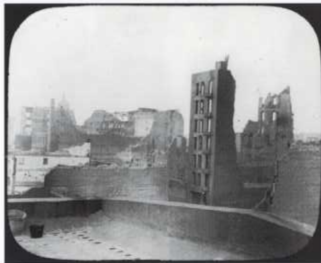
Destruction outside the San Francisco Mint after the 1906 earthquake and fire. RG 104
