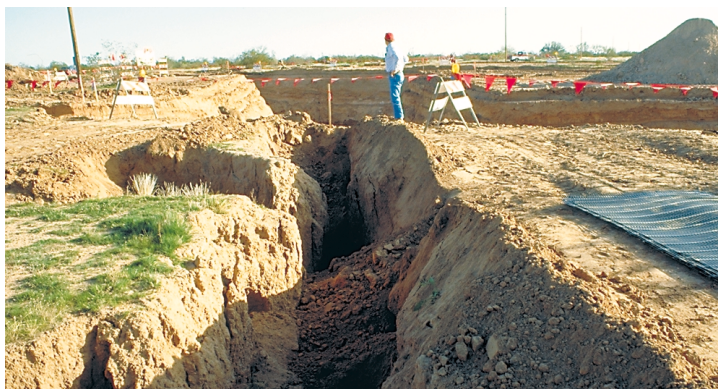
Part of this fissure south of Apache Junction has been trenched and backfilled for a land bridge.
