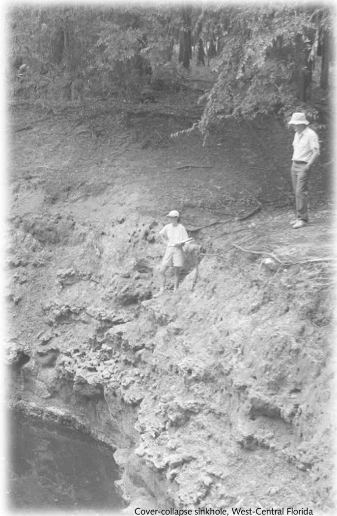
Cover-collapse sinkhole, West-Central Florida
