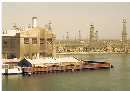
Oil and gas removal in Long Beach, California caused subsidence. Levees were built to prevent flooding of the oil fields and port facilities.
