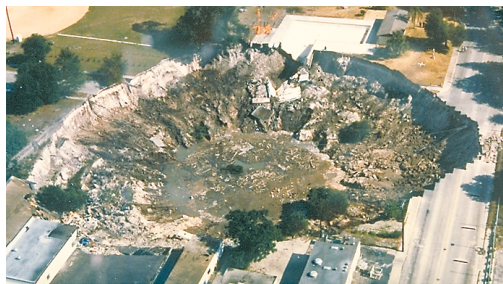
Cover-collapse sinkhole Winter Park, 1981
