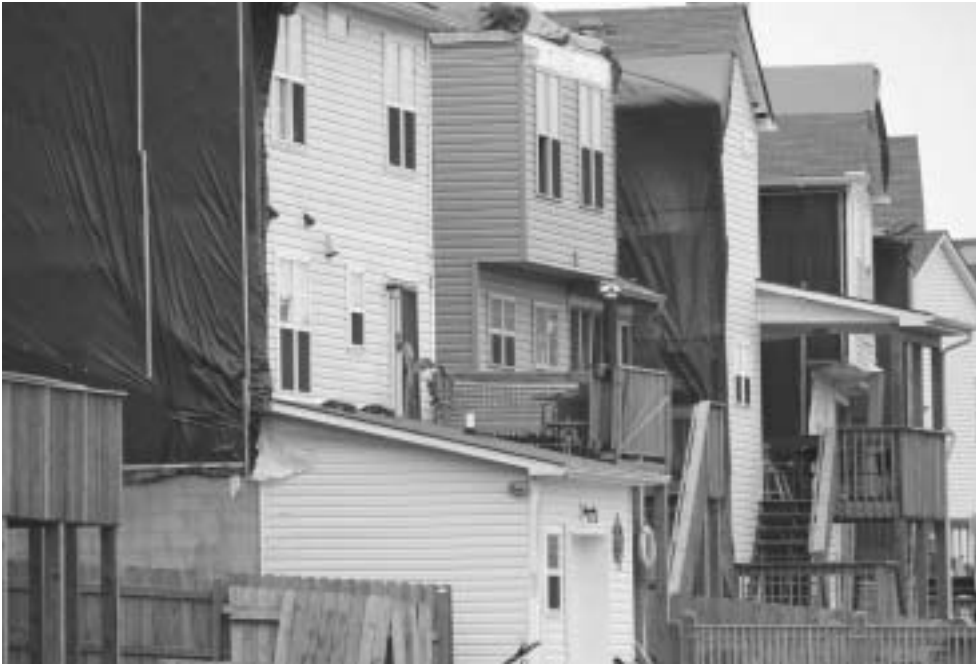
Houses damaged by a tornado are wrapped in plastic to keep water from damaging them further. Photo by Michael Rieger
