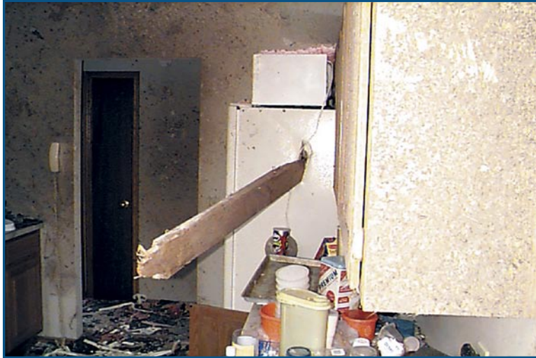
2" x 6" missile penetrating a refrigerator, Midwest Tornadoes of May 3, 1999
