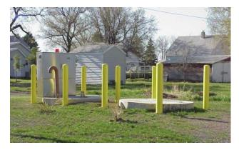
A new master lift station has been built away from the river in an area that now can be better protected from flooding. Removing the old lift station from the edge of the riverbank also enables the city to construct temporary dikes to keep floodwaters getting into town.
