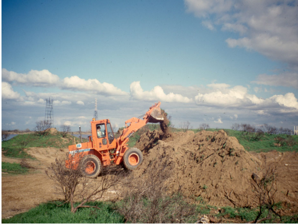
Constructing dunes using existing sand. USFWS Photo
