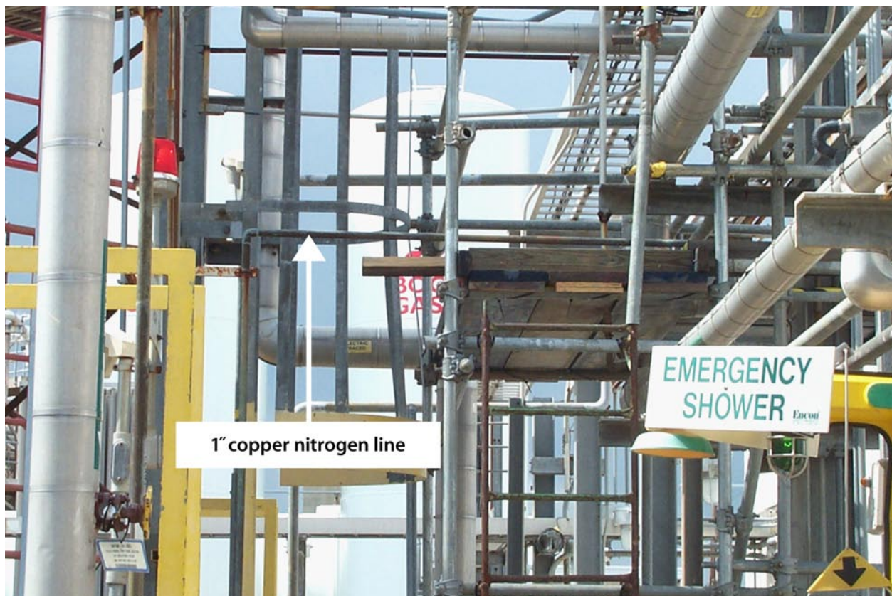
Figure 1-1. Scaffold and nitrogen line
