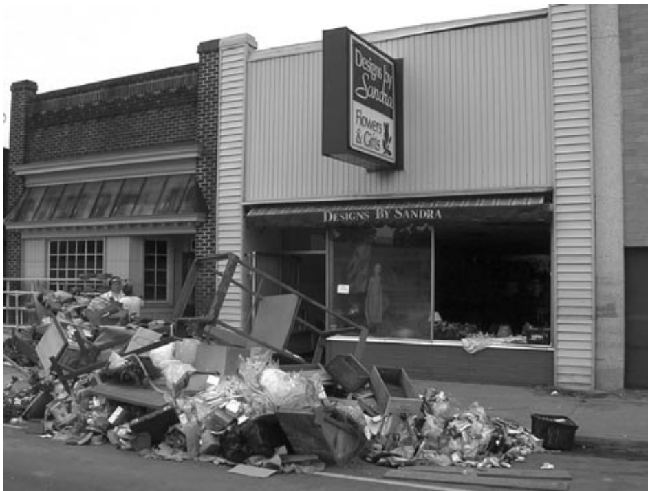
The windows of this store had not been boarded up, allowing hurricane winds to enter and do major damage inside the structure.
