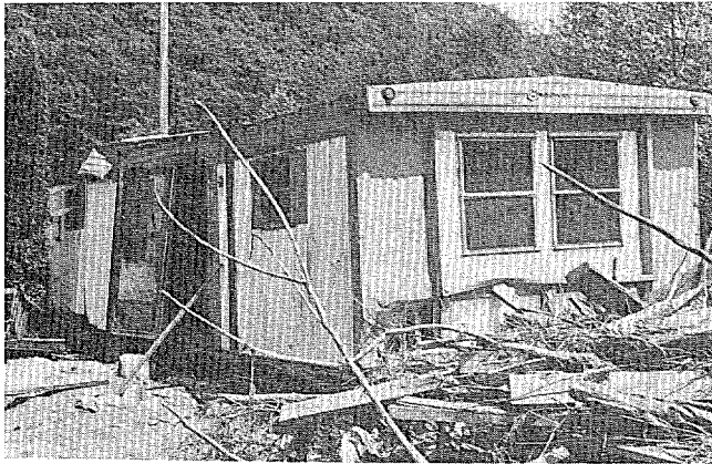
Figure 2.4 Damage From Debris
