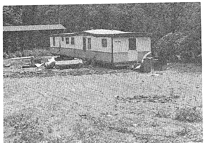
Figure 1.24 Shallow Flooding Damage
