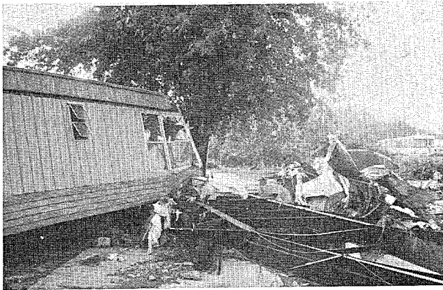
Figure 1.15 Movement From Foundation
