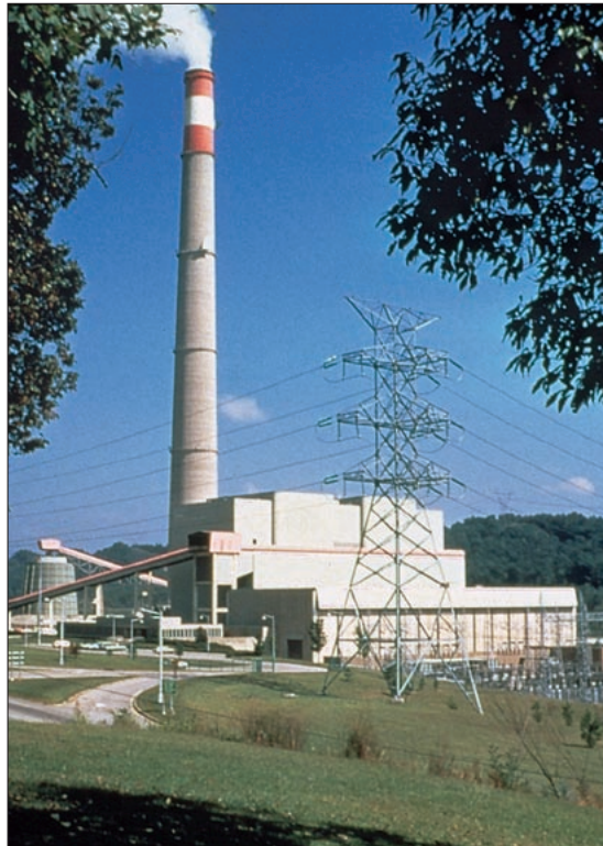
Bull Run thermoelectric power plant, Anderson County, Tennessee. (Photo courtesy of Tennessee Valley Authority.)
