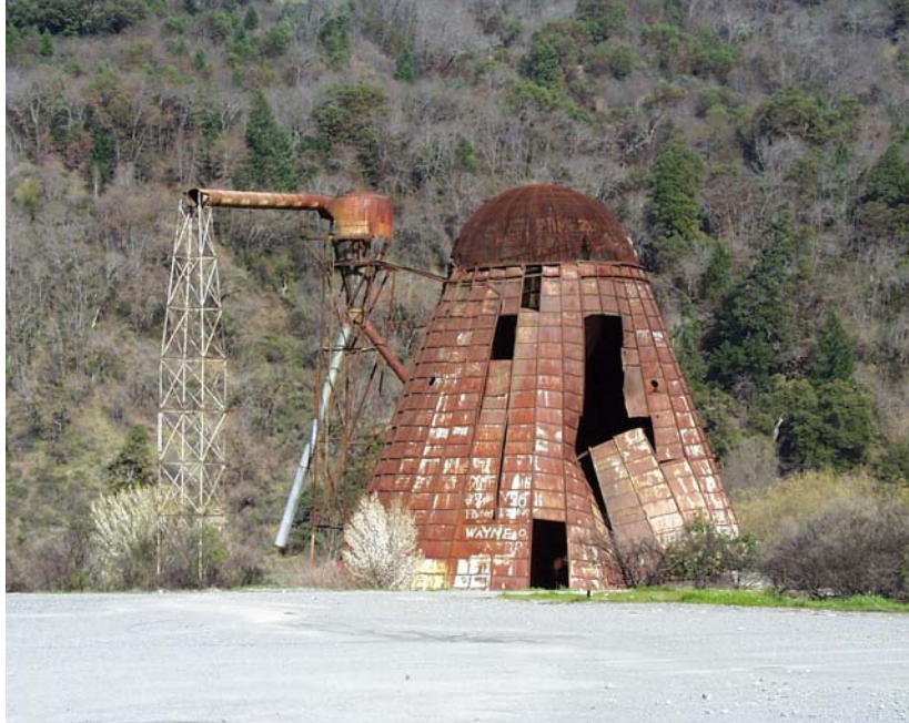
Tee-Pee Burner at Abandoned Cal-Pac Mill
