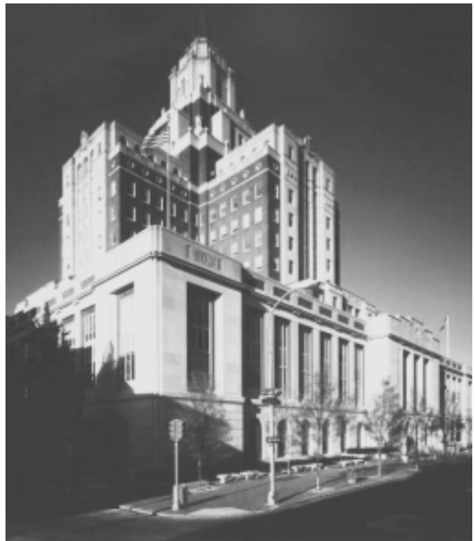
The U.S. Custom House in Philadelphia will receive numerous upgrades under a recently awarded $1.9 million Energy Savings Performance Contract.
