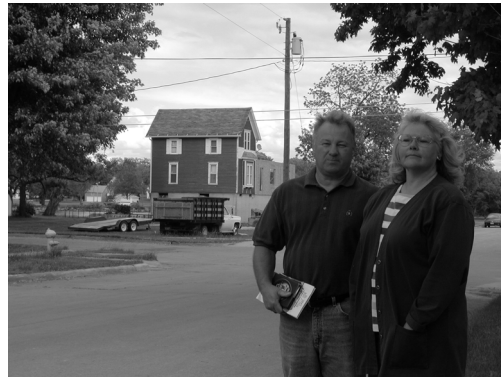
Bob and Joni Hocken decided that selling their Independence, Iowa, home of 27 years wasn't an option, even after it flooded twice in 1999. Instead, they elevated the home, seen in the background, so that the living areas are now well above the floodplain. (Photo: David Teska, FEMA)
