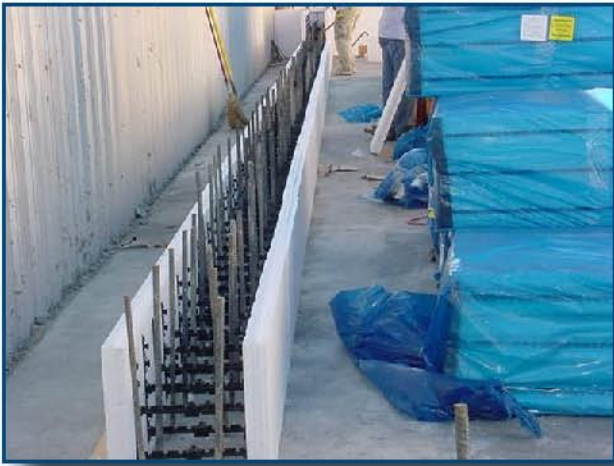
All perimeter walls were constructed with insulating concrete forms and reinforced with #5 bars spaced 8 inches on center to resist 250 mph wind speeds.
