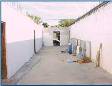
Interior of shelter, showing insulating concrete form perimeter walls.
