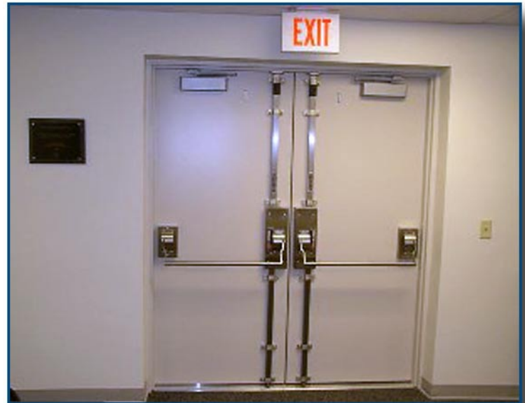
View of the FEMA 361-compliant double door with 3-point latching hardware from inside shelter.
