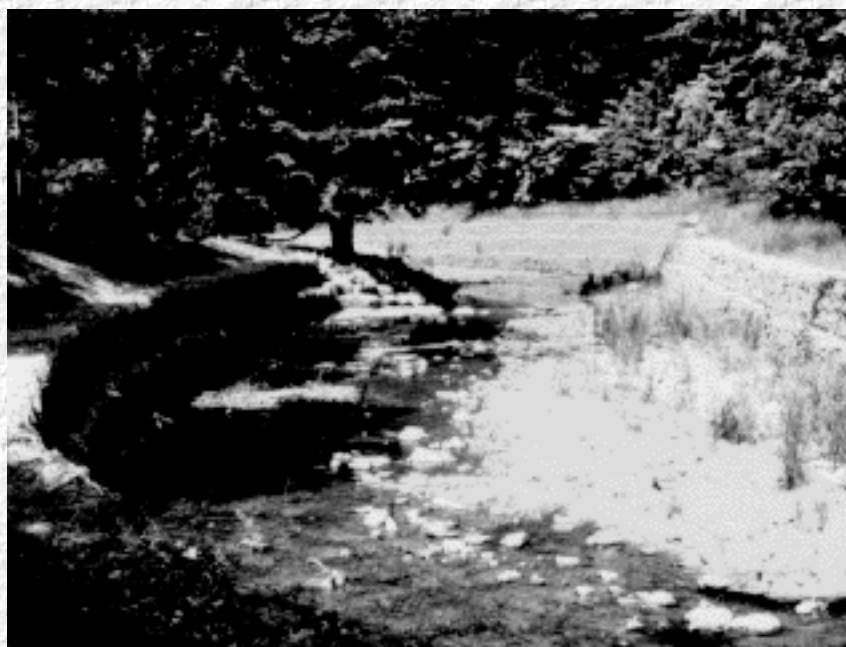
Figure 10. Gabion Basket Revetment
