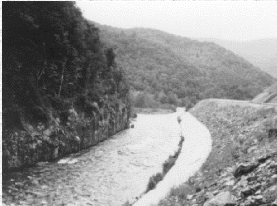
Figure 13. Concrete Pavement Revetment
