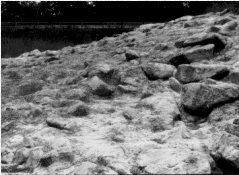
Figure 12. Grouted Riprap
