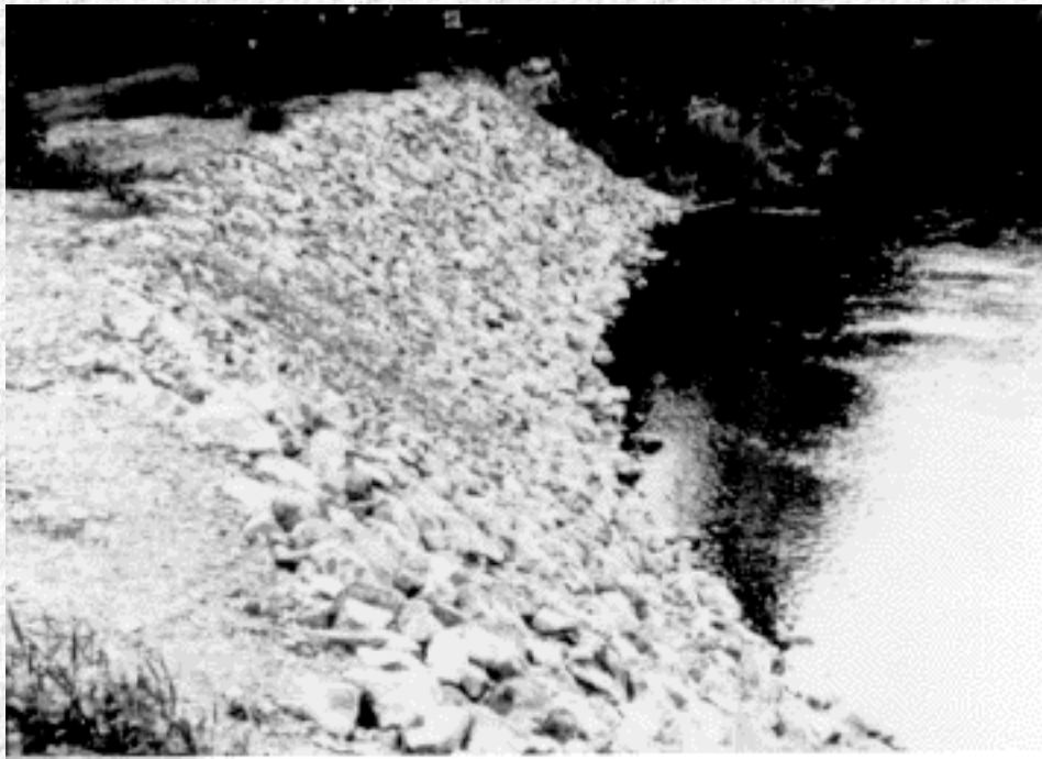
Figure 6. Hand-placed Riprap
