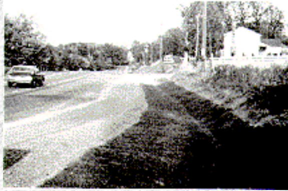
Figure 3. Vegetative Channel Lining (class D retardance)
