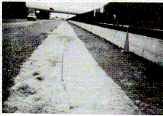
Figure 14. Installed Curled Wood Mat Channel Lining
