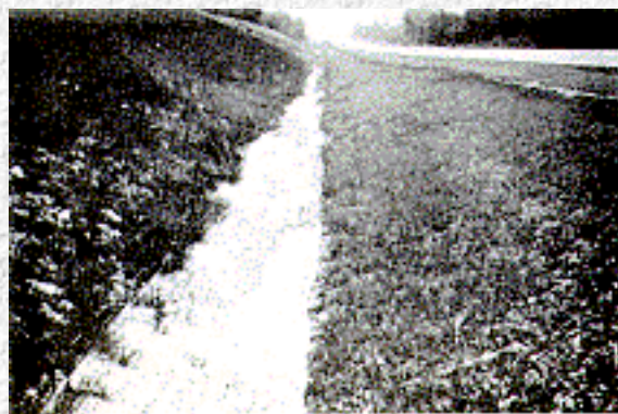
Figure 10. Installed Jute Net Channel Lining
