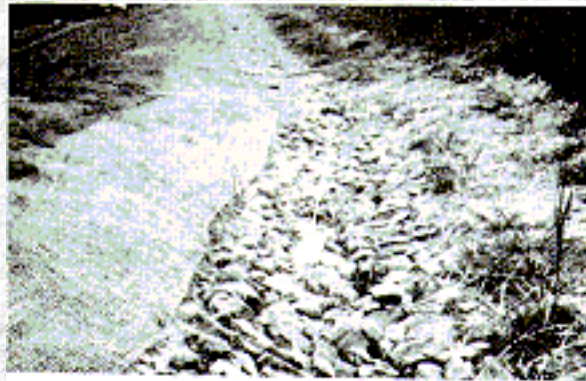
Figure 2. Composite Channel Lining (riprap and jute net)
