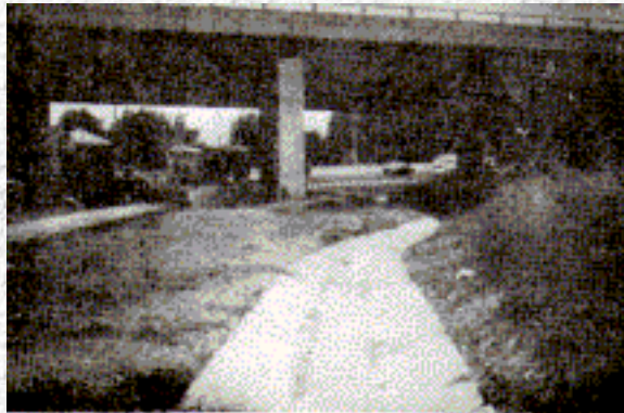
Figure 1. Rigid Concrete Channel Lining
