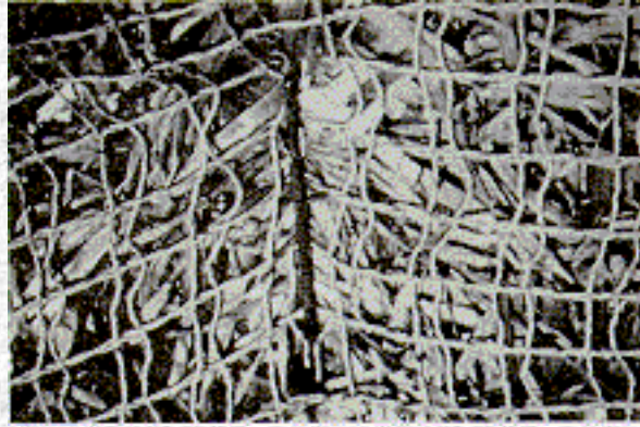
Figure 17. Straw With Net Channel Lining
