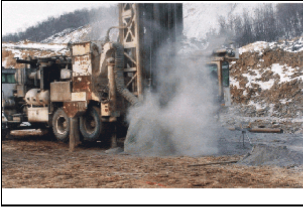
Cooperative research effort to lower surface drill operator silica dust exposure by improving cab filtration efficiency and pressurization.
