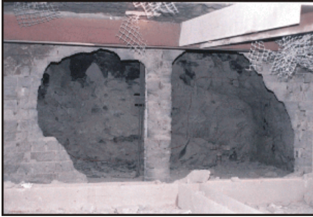
Remains of standard seal destroyed by methane-air-oxygen explosion.
