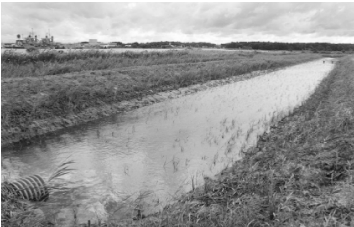
Constructed wetland at Little Creek Naval Amphibious Base, VA
