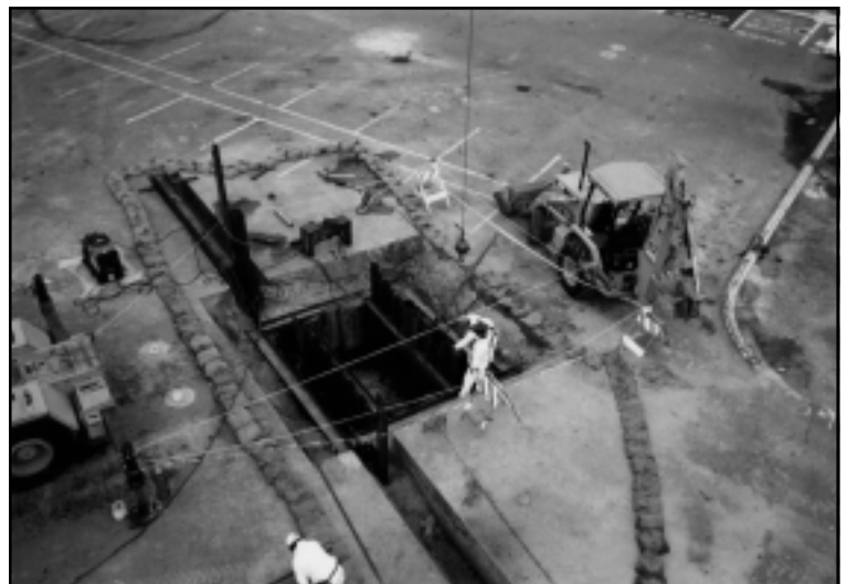
Figure 1 - Construction of funnel-and-gate system at Moffett Field
