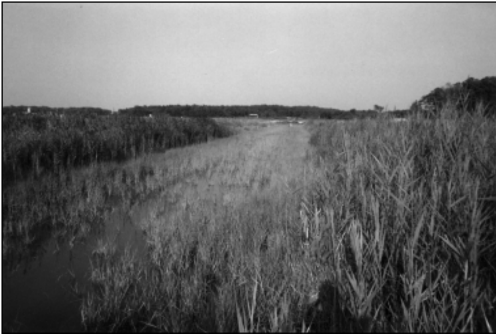
Figure 3 - Constructed wetland at Little Creek Naval Amphibious Base, VA.
