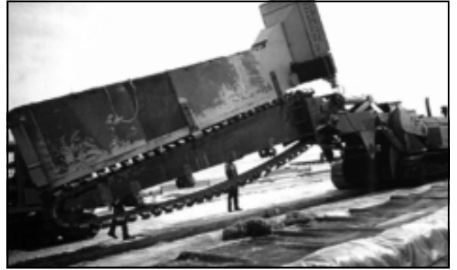
Figure 3 - Specialized "track type" trencher with hopper for reactive media.
