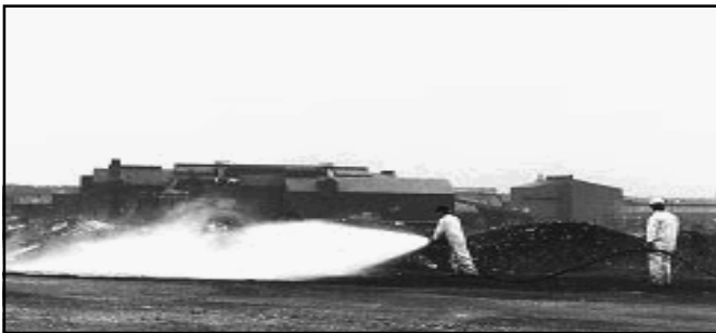
Figure 2. Applying SOIL-SEMENT® to a soil pile.
