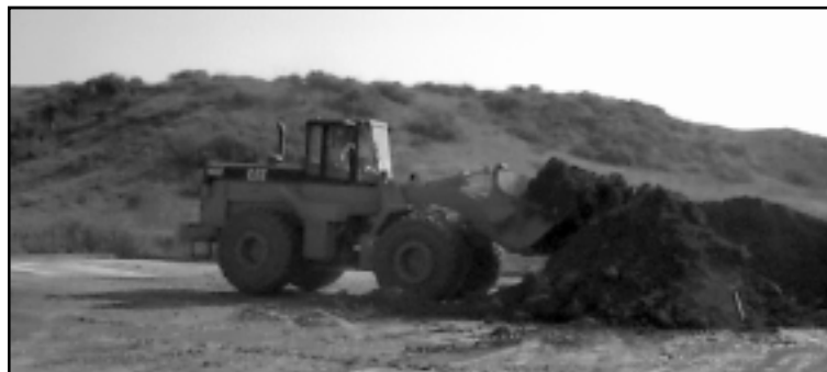
Figure 4. Removal of treated soil.
