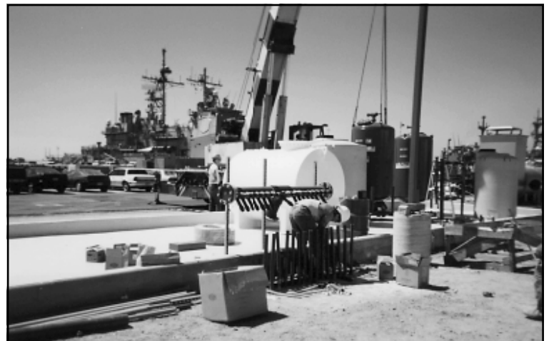
Figure 1. Extraction and Treatment System Installation
