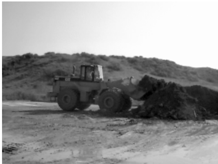
Figure 4. Removal of treated soil.
