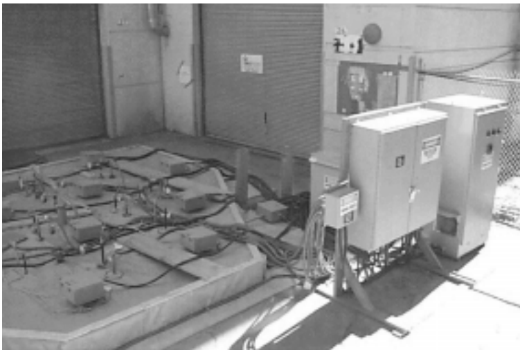
Thermal well treatment area
