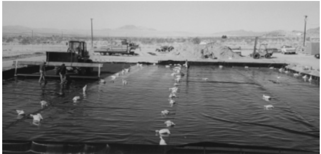
Figure 1. Liner installation
