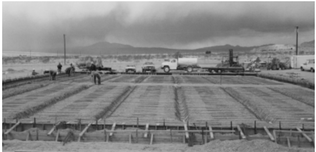
Figure 2. Rebar installation
