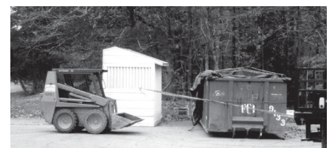
Figure 2. Rolloff box containing Investigation Derived Waste (IDW).
