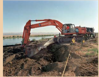
Removing contaminated soil near the retired reactor areas along the Columbia River
