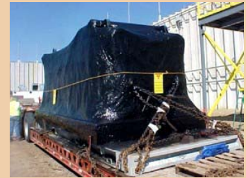
ALARA concept – use of Instacote™ instead of size reduction or cutting
