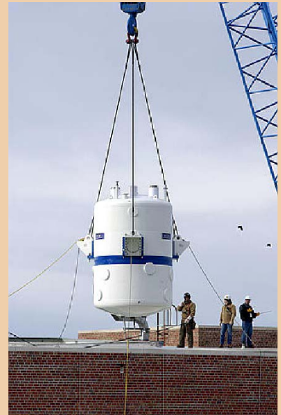
A powerful magnet being lifted by crane at Pacific Northwest National Laboratory
