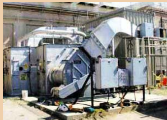
Rocky Flats workers remove the exterior plenum outside Building 444
