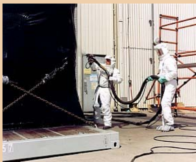
Workers apply polyurea coating to equipment at Rocky Flats
