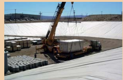
Treated, mixed low-level waste is disposed of in RCRA-compliant landfills such as this one at Hanford
