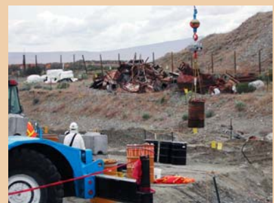
A drum is moved from the Hanford 618-4 burial ground to be overpacked
