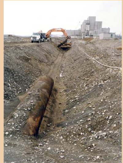
Digging up reactor effluent cooling water piping and surrounding contaminated soil
