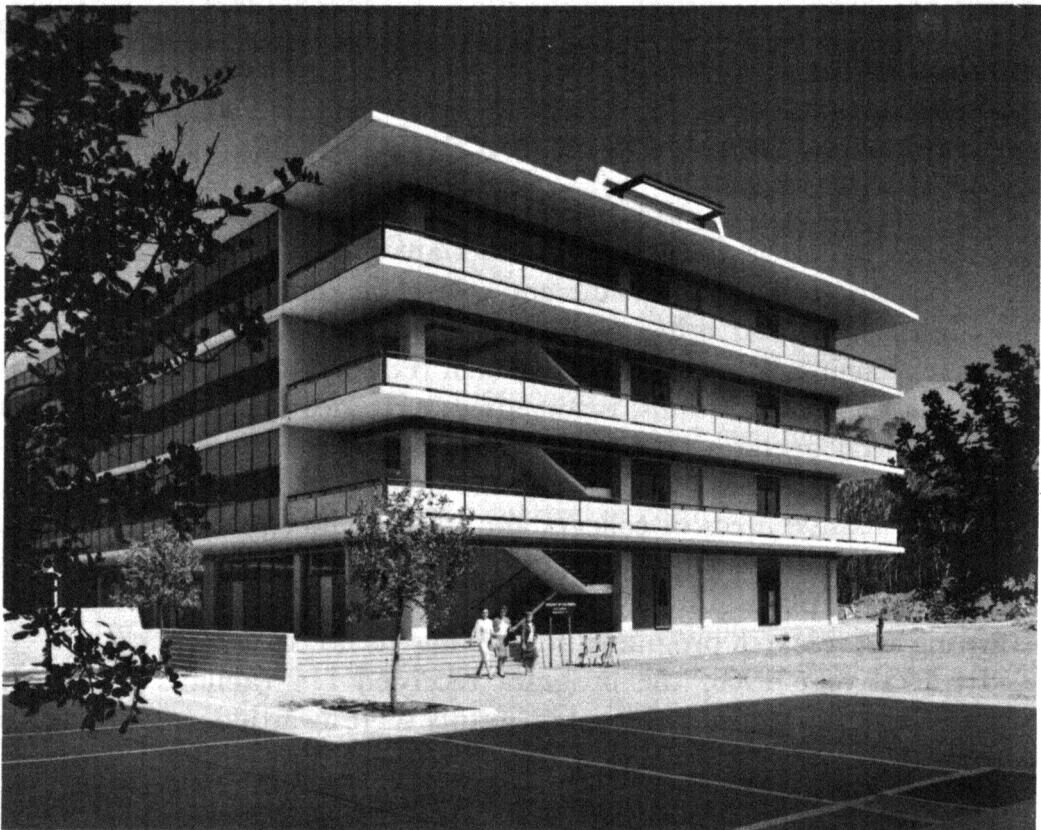
Figure 34. — Building C of Revelle College, University of California, San Diego.
