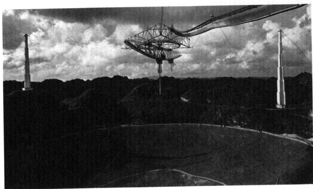
This view of the Arecibo installation shows two of the three towers supporting the feed support structure 435 feet above the spherical mesh reflector. (Photo Cornell University)
