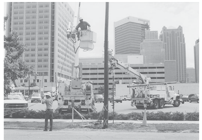
Line installers work on both telecommunications and electrical lines.
