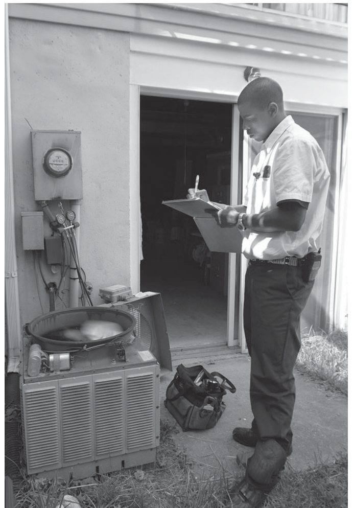
Service contracts—which involve heating, air-conditioning, and refrigeration maintenance on a regular basis—are becoming more common.
