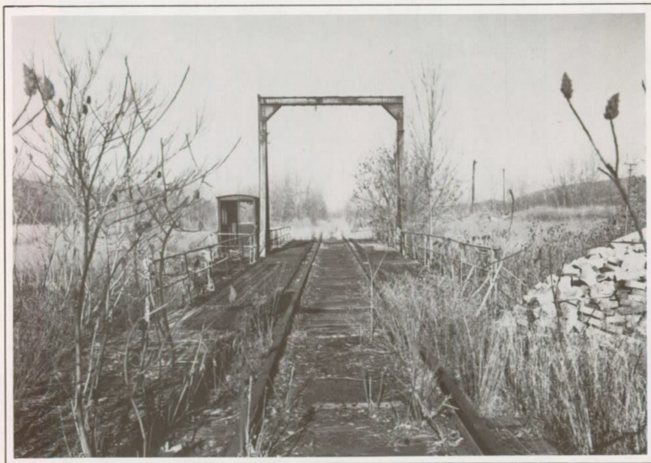
Illustration 14. East Altoona Shops, Turntable (Ca. 1903), Served the Great East Altoona Roundhouse (Roundhouse Demolished Ca. 1956). Photograph by Jack E. Boucher, 1988. Courtesy of Historic American Engineering Record, Washington D. C.
