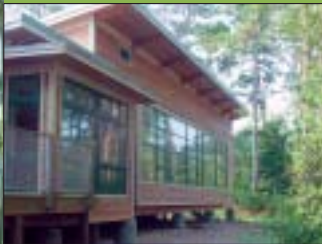
The indoor environment is enhanced further through abundant daylight and fresh air ventilation.
