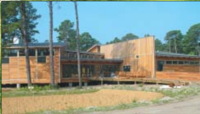
The Center uses an innovative constructed wetlands wastewater treatment system. The system includes a primary clarifier, a subsurface-flow-constructed-wetland with recycle, and a re-circulating sand filter. The effluent is used to flush toilets.
