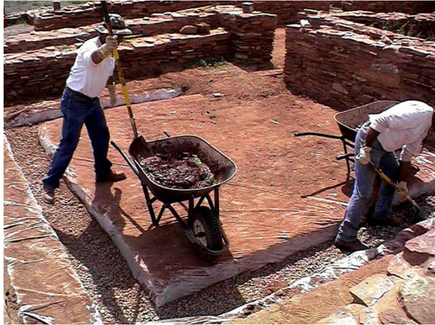
Salinas Pueblo Missions National Monument preservation crew repairing drains.
