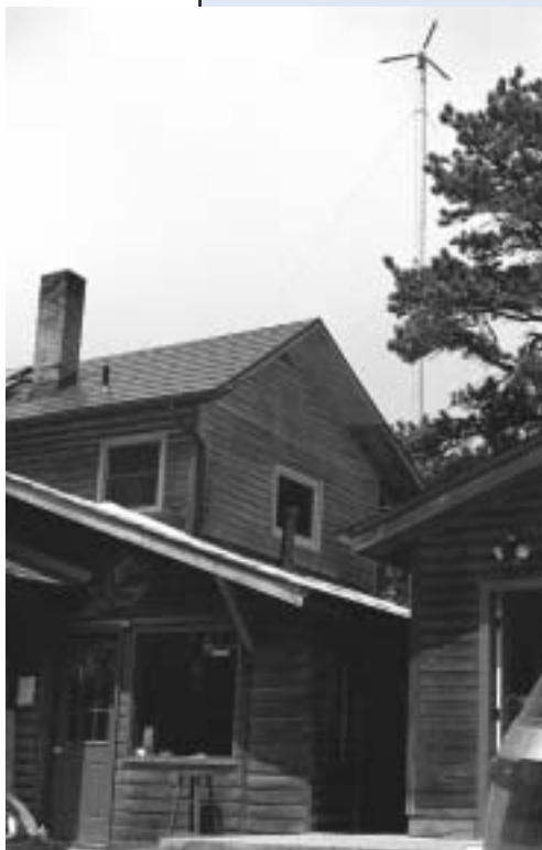
Jim Green, NREL / P1A12796
