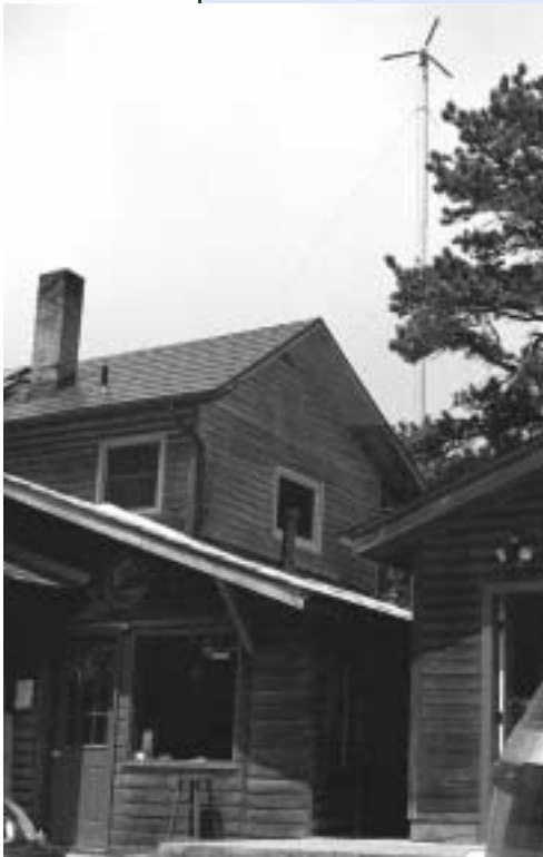
Jim Green, NREL / P1A12796
