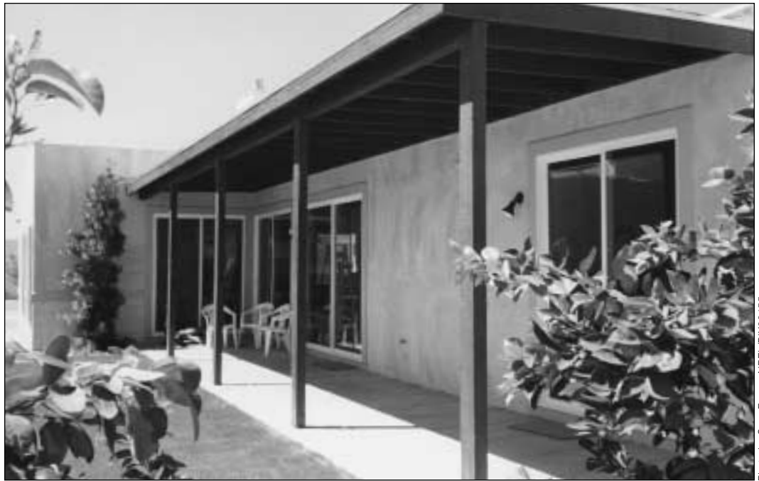
This house in Arizona features a passive solar design with overhangs above the south facing windows.
