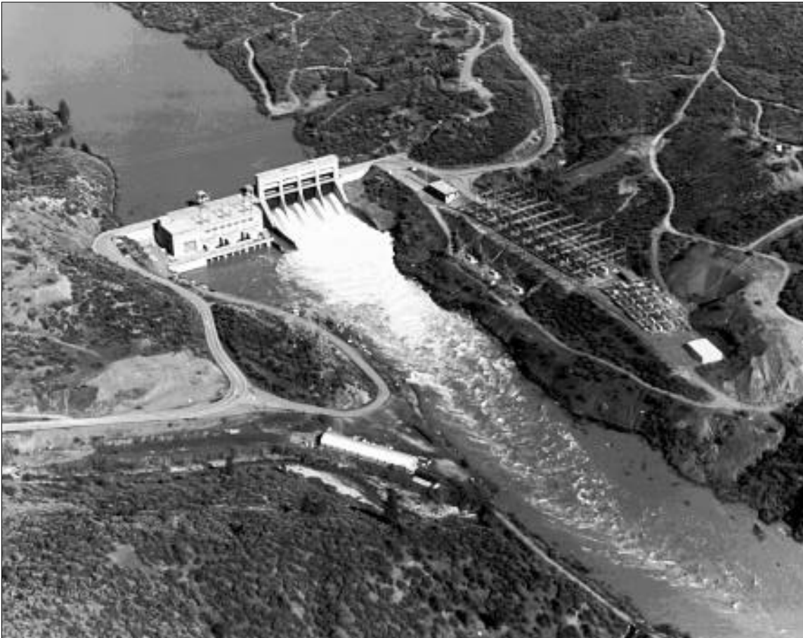
This hydropower plant is located at the Keswick Dam on the Sacramento River north of Redding, California.
