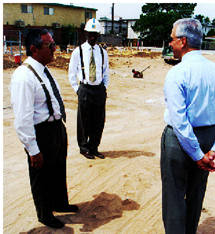
ASVET Frederico Juarbe Jr. with staff from Rehabilitation Services and Veterans Programs at the site of an 18-unit apartment complex for disabled veterans.
