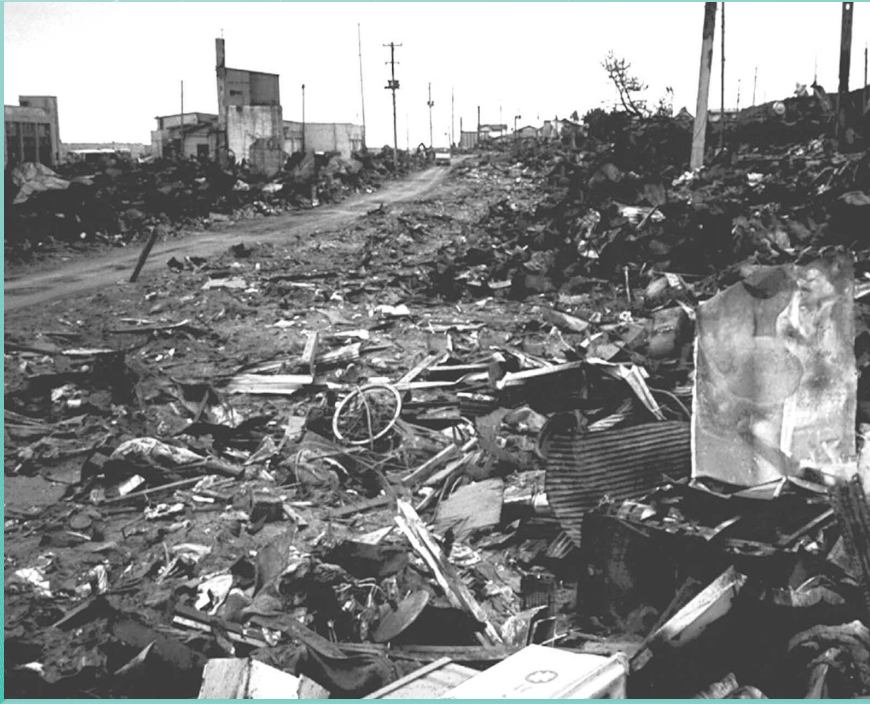
Aonae, Okushiri Island, Japan. Total destruction of houses and other buildings resulting from the tsunami of July 12, 1993, in the Sea of Japan. Numerous fires broke out following the tsunami adding to the property loss and misery. Over 120 people were killed by the tsunami in Japan.
