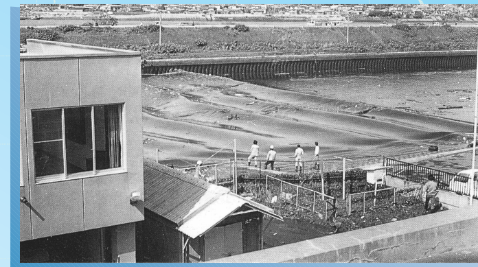
Noshiro, Harbor, Japan. May 26, 1983 Japan Sea earthquake. The tsunami, upon entering a waterway, generated a continuous train of short-period waves. (Tokai Univ. report)
