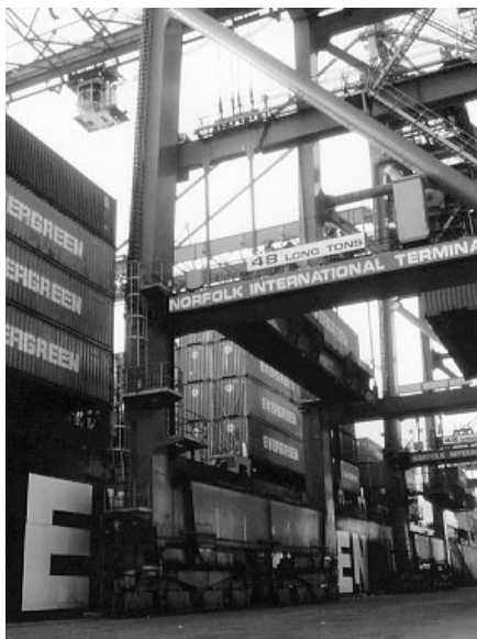
Virginia Port Authority
