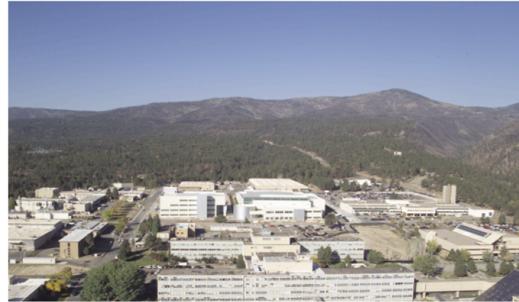
Overview of the main Los Alamos National Laboratory technical and administrative site on the Pajarito Plateau looking west toward the Jemez Mountains.
