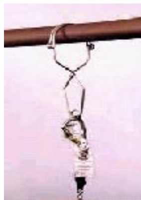
Figure 3-1. A spring-loaded wire form anchorage connector
