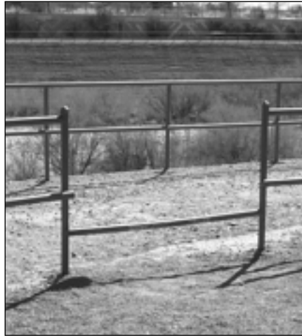
Trail managers along the Santa Cruz River in Tucson use a number of gates with a bar one foot off the ground to deter ATVs. Joggers with strollers are able to cross the bars with ease while ATVs and motorcycles must be carried over.
